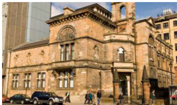
Anderson College building (built 1889), Glasgow University
